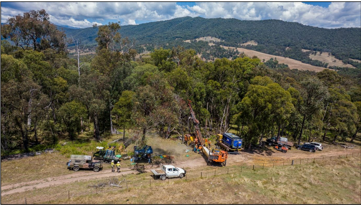
Figure 4 – Drilling of EMRC07 at Granite Flat.
