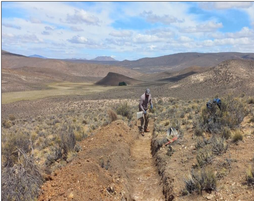
Figure 6: Example of shallow hand dug trench
