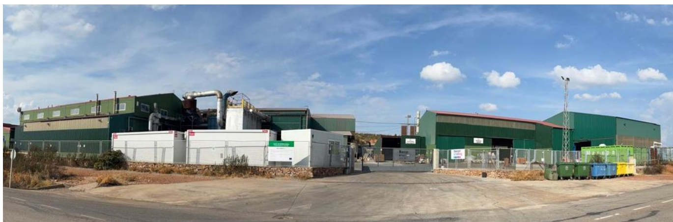
Figure 3. External view of the Robledollano Tin Smelter, owned by Iberian Smelting S.L
