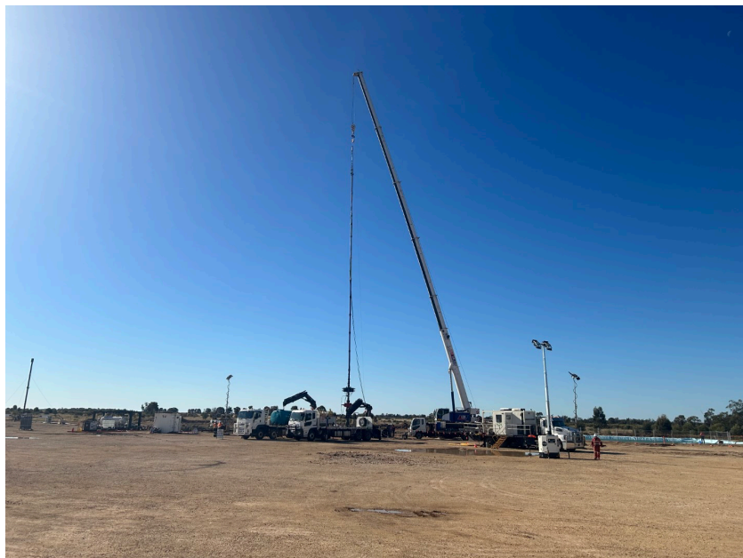
Wireline rigged up on Daydream 2
