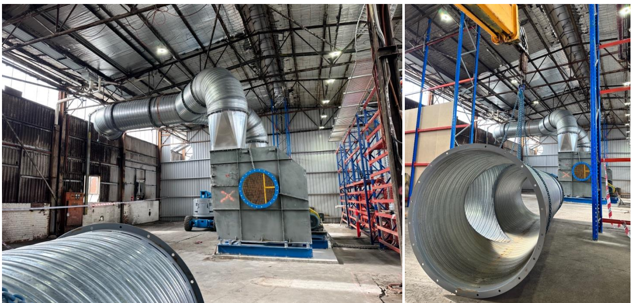
Photos (above): The ground level of the building is being prepared to receive several megawatts of servers, which will be mounted on racks. Fans will draw the waste heat from the enclosed data centre to the conditioning system and Packed Bed Dryer.
