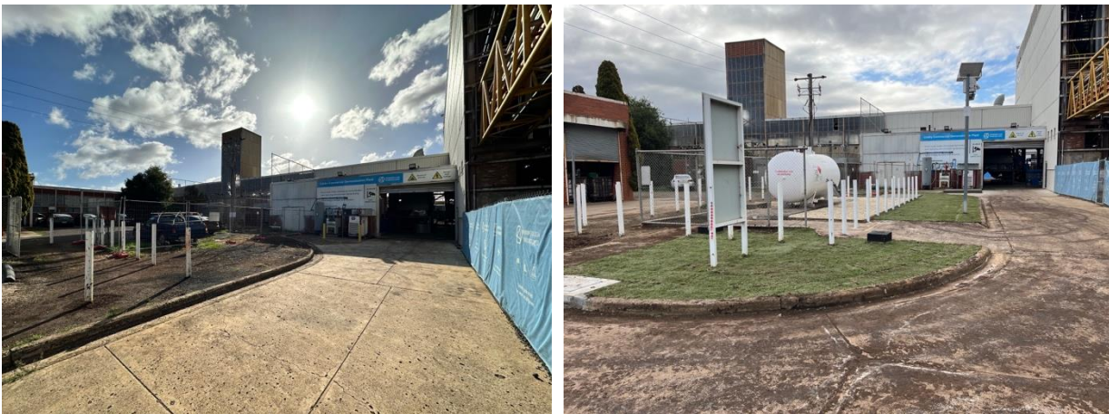
Photos (above): Before (left) and after (right), the preparation of the site for the installation of the Panasonic H2 Fuel Cell adjacent to the existing COLDry demonstration plant and LPG vessel.
