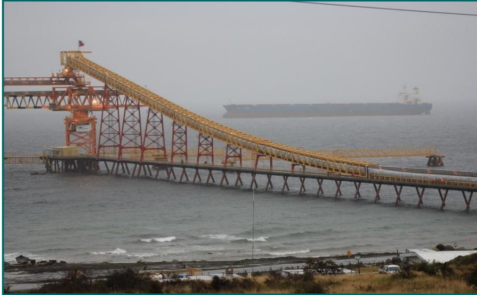
Photo 1. Ship Loader at Mina Invierno
