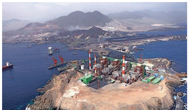
Photo 2. Guacolda coal fired power station in Region III (600MW) is one of Chile's 12 existing coal fired power stations
