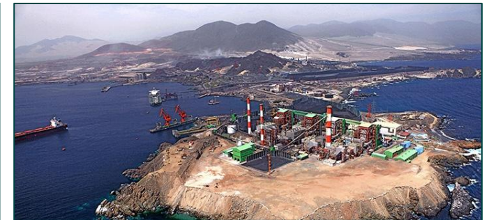
Guacolda Coal Fired Power Station Region III (600MW)
