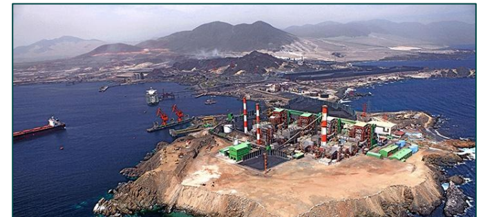
Guacolda Coal Fired Power Plant Region III (600MW)
