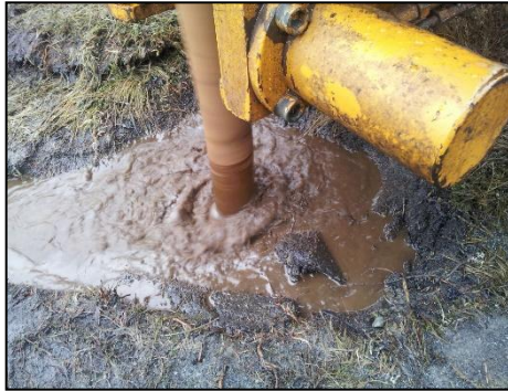
Brown drill water indicative of coal being drilled
