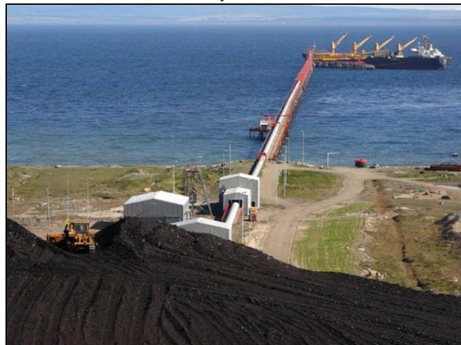
Photo 1. Panamax ship loader at Puerto Pecket
