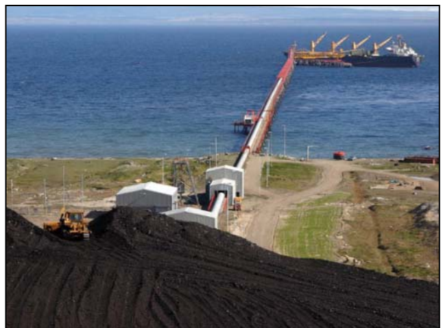
Photo 5. Panamax ship loader at Port Pecket
