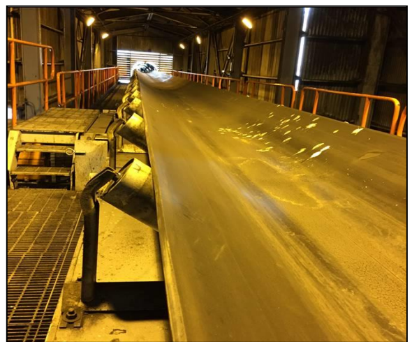
Photo 9. Idle conveyor system
