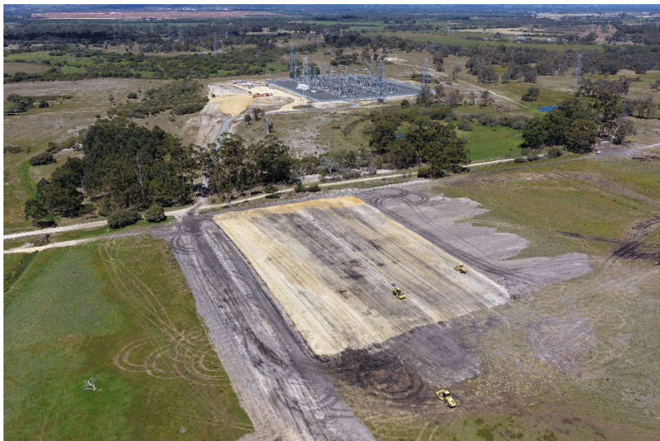
Image 2. Preparation of pad for Frontier substation
