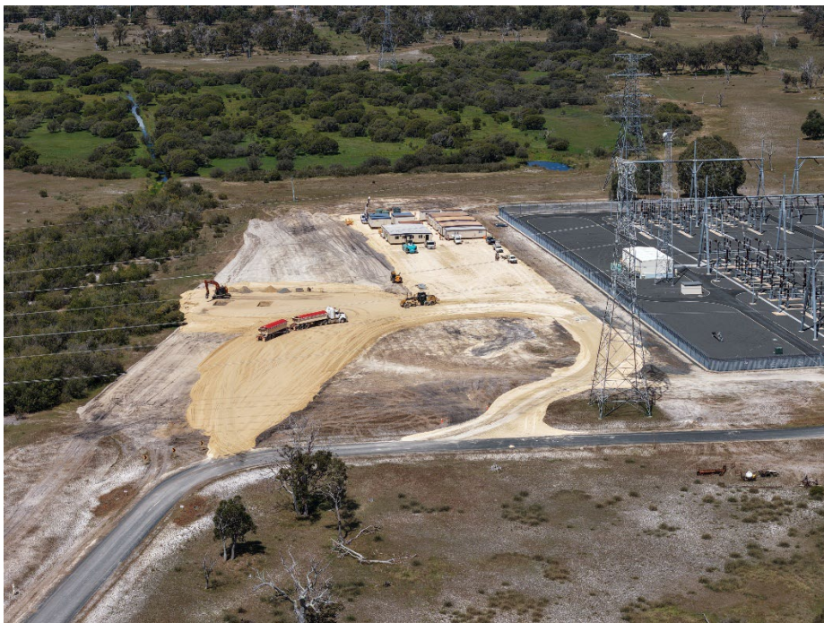
Image 4. Monford administration offices adjacent to the Landwehr Terminal
