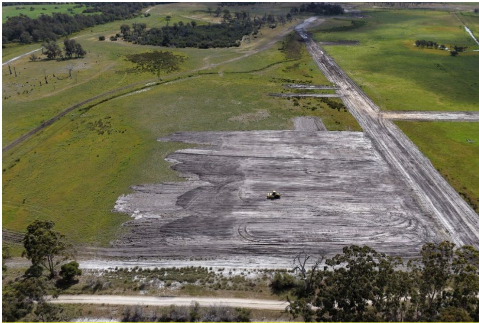
Image 1. Site preparation works
