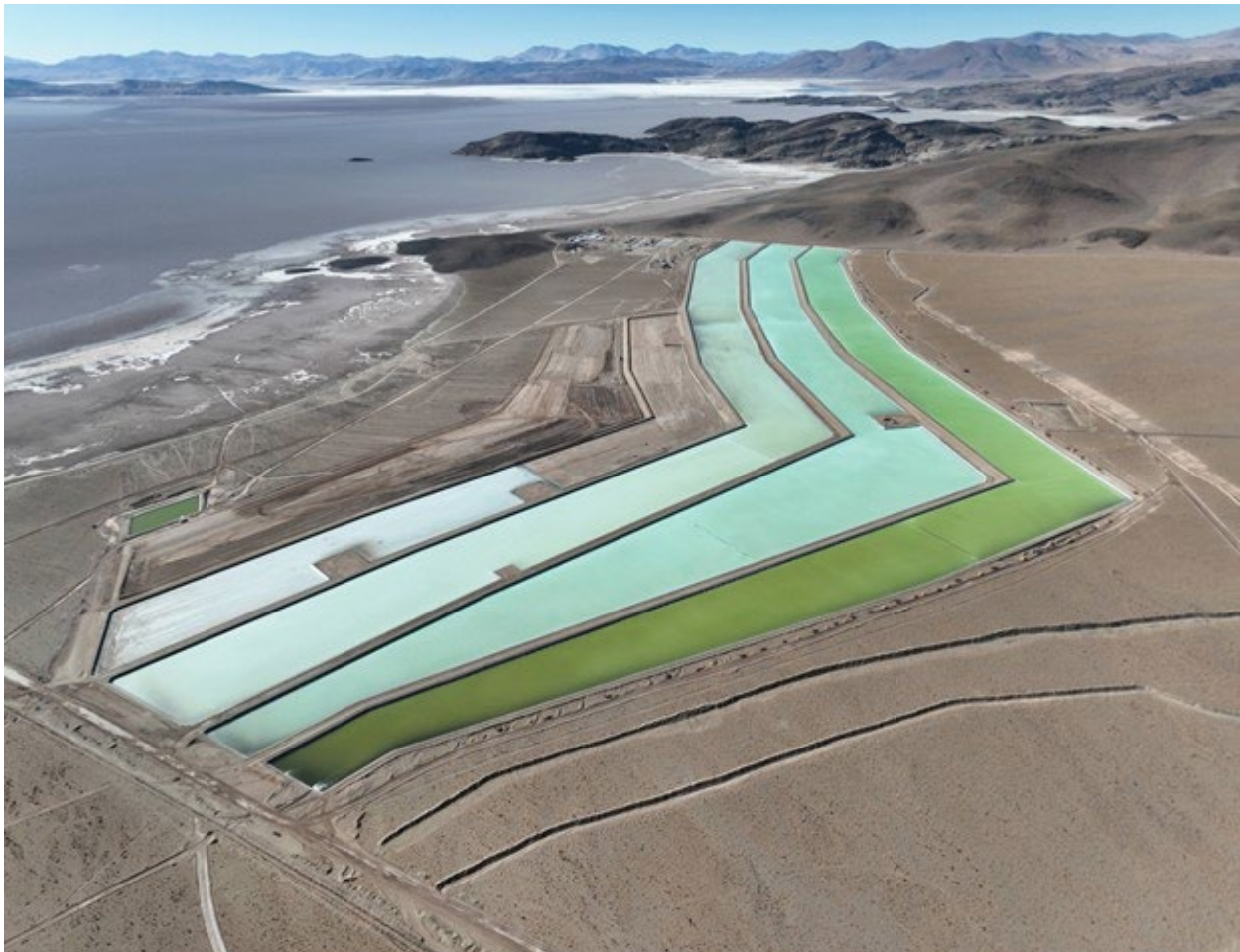
HMW Project looking south
