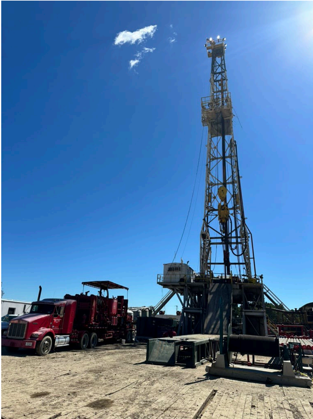
Figure 1: Drilling rig and service equipment at the Zydeco-1 well site.
