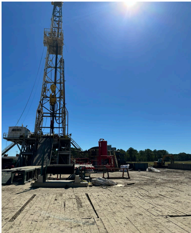
Figure 4: Drilling rig and equipment at the well site.
