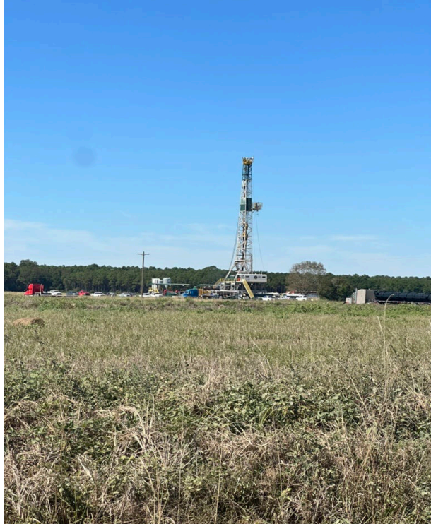
Figure 2: View of the drilling location from the surrounding field
