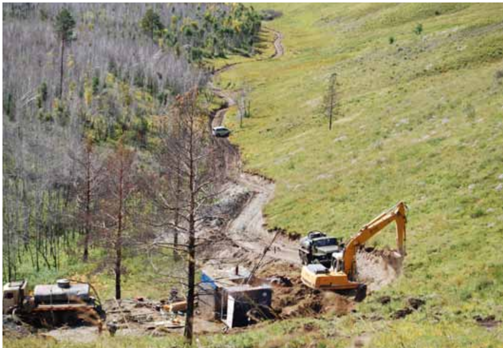
Figure 4-6: Trenching at the Huiten Gol Prospect
