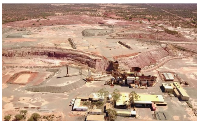
Extensive Site Infrastructure including 600,000tpa processing plant
