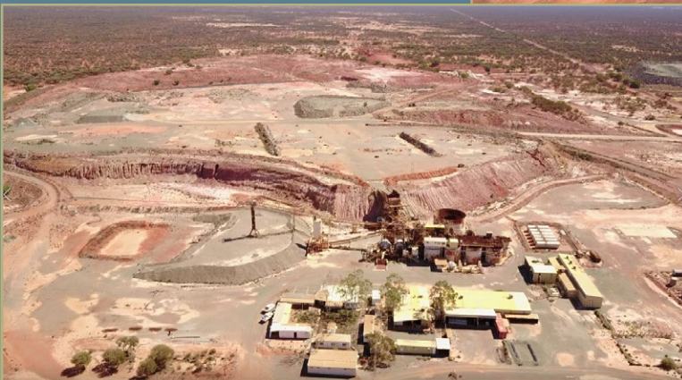
Extensive Site Infrastructure including 600,000tpa processing plant
