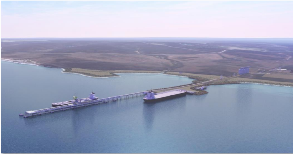
Figure 1 – Stage I development at Cape Hardy envisages a jetty and wharf structure suitable for Panamax-class vessels and includes a tug jetty and causeway.
