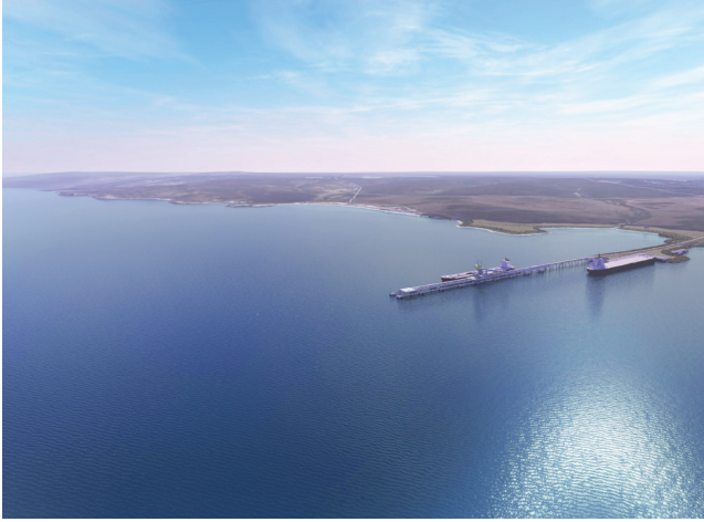
Cape Hardy Stage I and II port precinct with initial Panamax berth and infrastructure mainly for grain export and later Capesize berths with infrastructure for bulk commodity minerals, green manufacturing and the import and export of other goods
