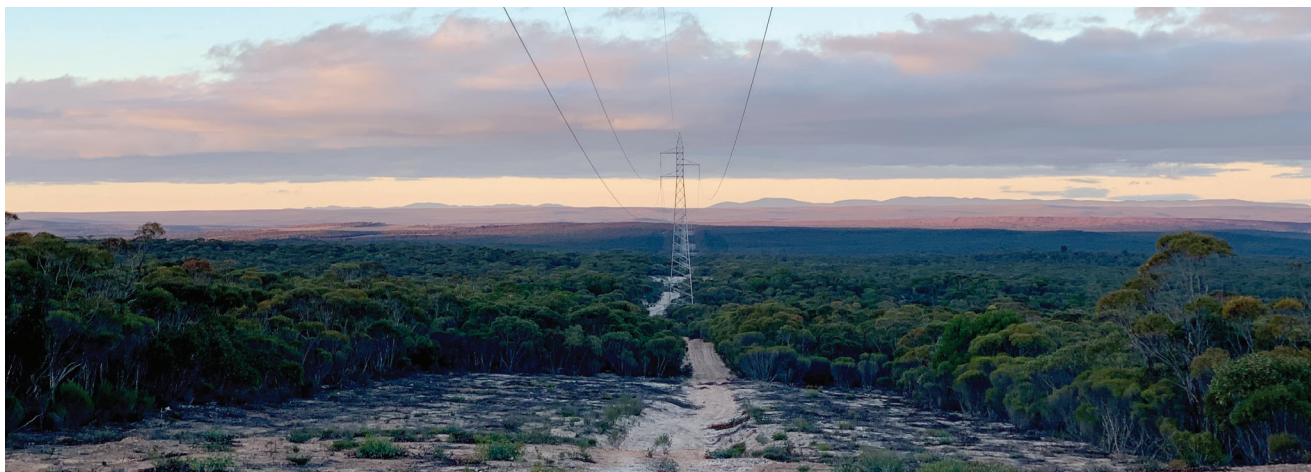
The Eyre Peninsula Link comprises a new 270 kilometre, high-voltage transmission line to be constructed from Cultana to Port Lincoln, via Yadrarie (Image- Jon Mussared)
