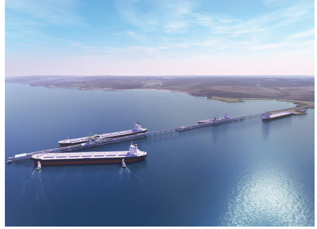
Cape Hardy Stage I and II port precinct with initial Panamax berth and infrastructure mainly for grain export and later Capesize berths with infrastructure for bulk commodity minerals, green manufacturing and the import and export of other goods
