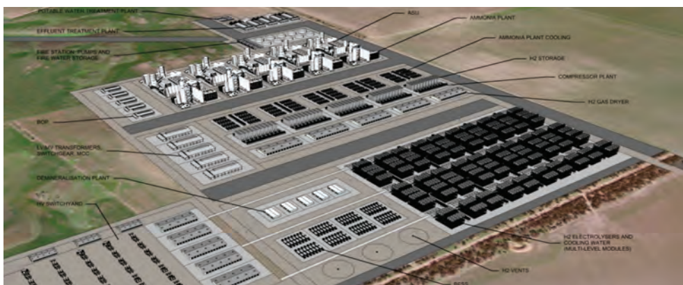
Key plant building blocks, Cape Hardy 5GW green hydrogen / ammonia production (courtesy of Amp Energy).
