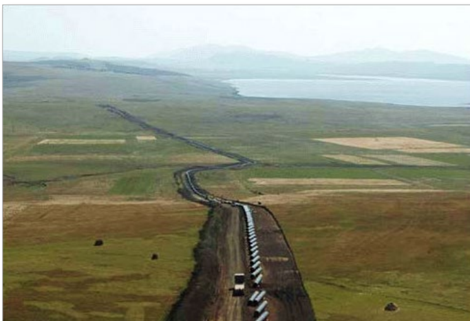
Pipeline construction within terrain similar to that traversed by the CEIP infrastructure corridor on the Eyre Peninsula. (Image: WSP Australia)
