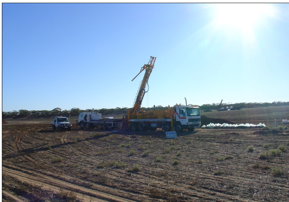
Figure 1 - Stage II drilling successfully completed during the Quarter
