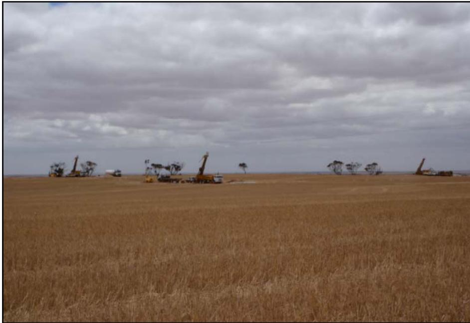
**Figure 2 – Drilling at the Warrambo Project is being undertaken by one RC drill rig (for pre-collars) and two diamond drilling rigs (for diamond tails).**
