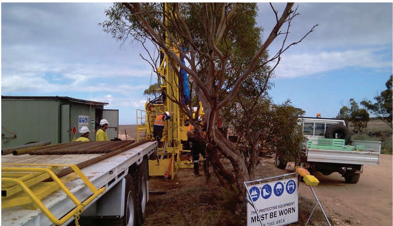
Figure 3. Geotechnical drilling in a road reserve at the CEIP.
