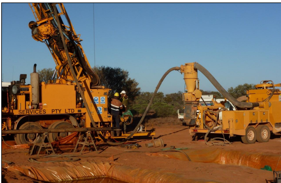
Figure 18 Stage III drilling utilises a UTR1200 multi-purpose drill rig.
