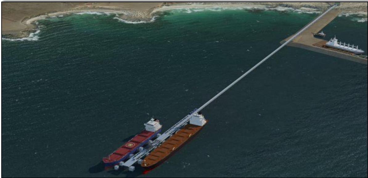
Rendering of Iron Road’s port proposal, Cape Hardy, showing jetty, wharf and module offloading facility (MOF).
