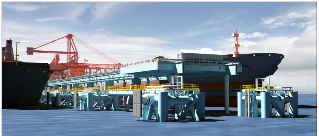
Figure 5: Rendering showing Cape Hardy wharf, with dolphins and shiploader.
