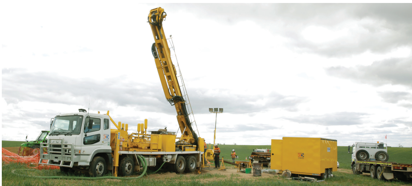
Drilling Programme at Warrambo, South Australia
