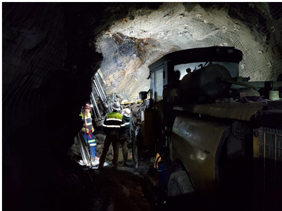
Progressing underground development works
