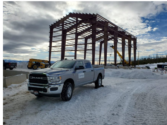
Flotation building progress
