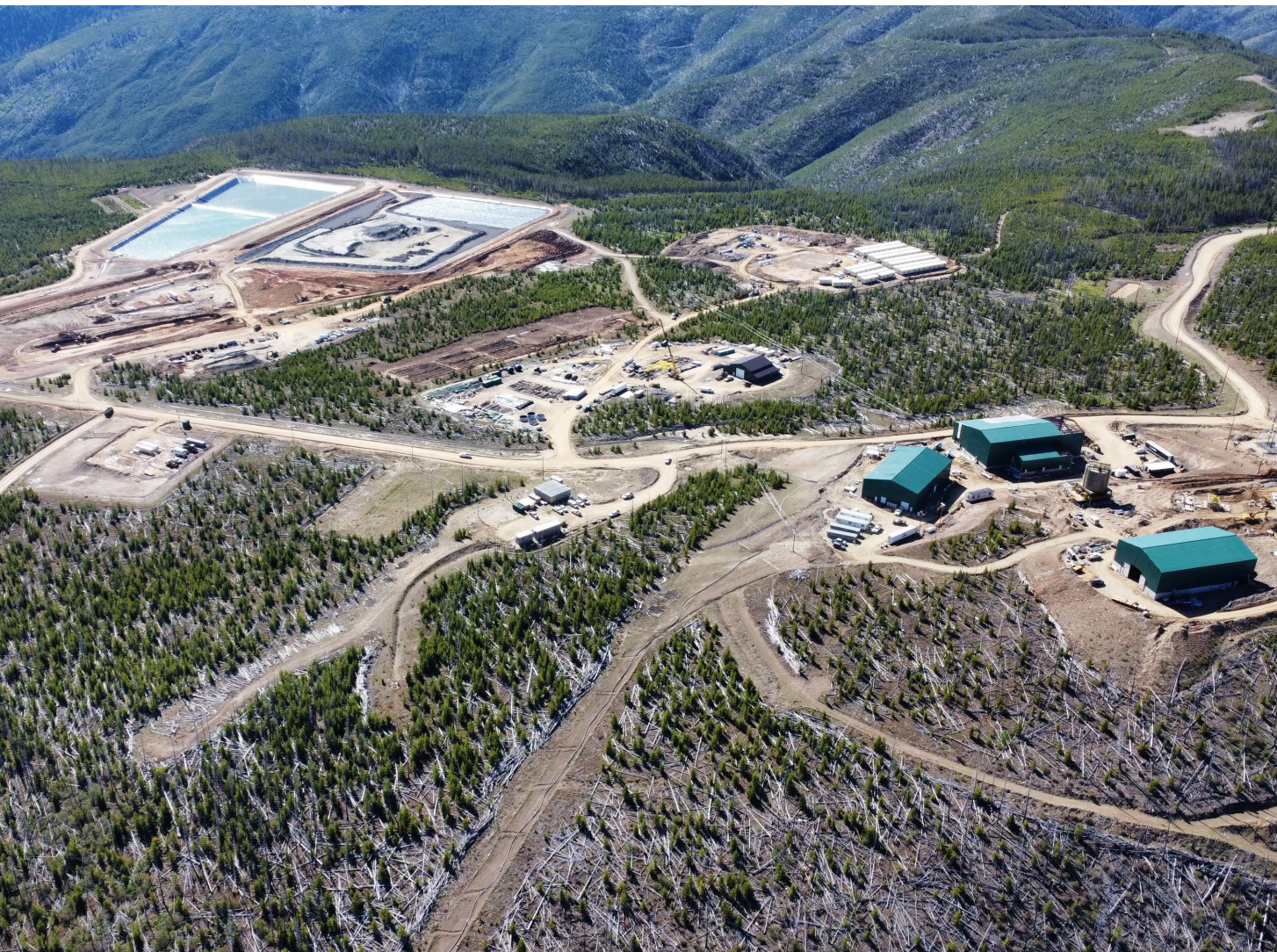
Surface construction at ICO (June 2022)
