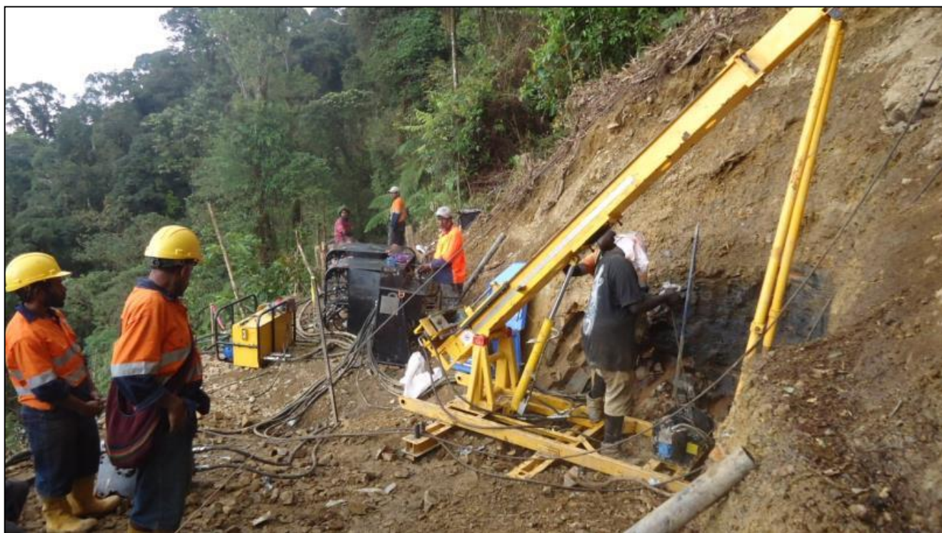
Photo 1. The CSD500 drill rig being set up on pad 1.
