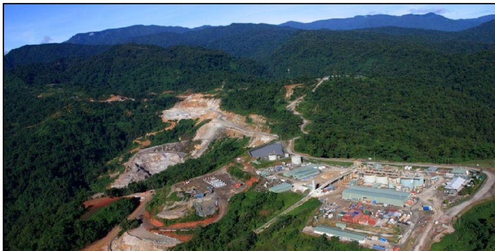
The Gold Ridge Mine processing plant and open pits (St Barbara photo looking south).
