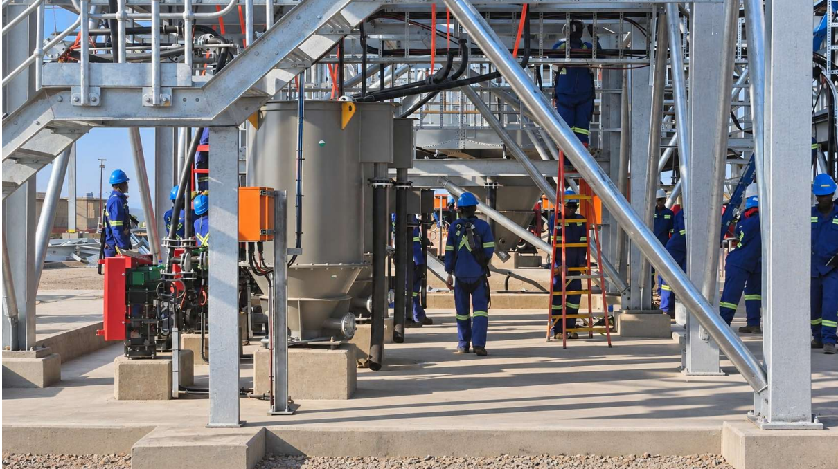
Picture 3. Kangankunde team undertaking installation works at the process plant
