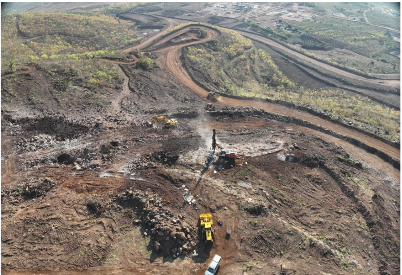
Picture 3. Development of upper pit access ramp, drilling activities and completed haul road at Kangankunde
