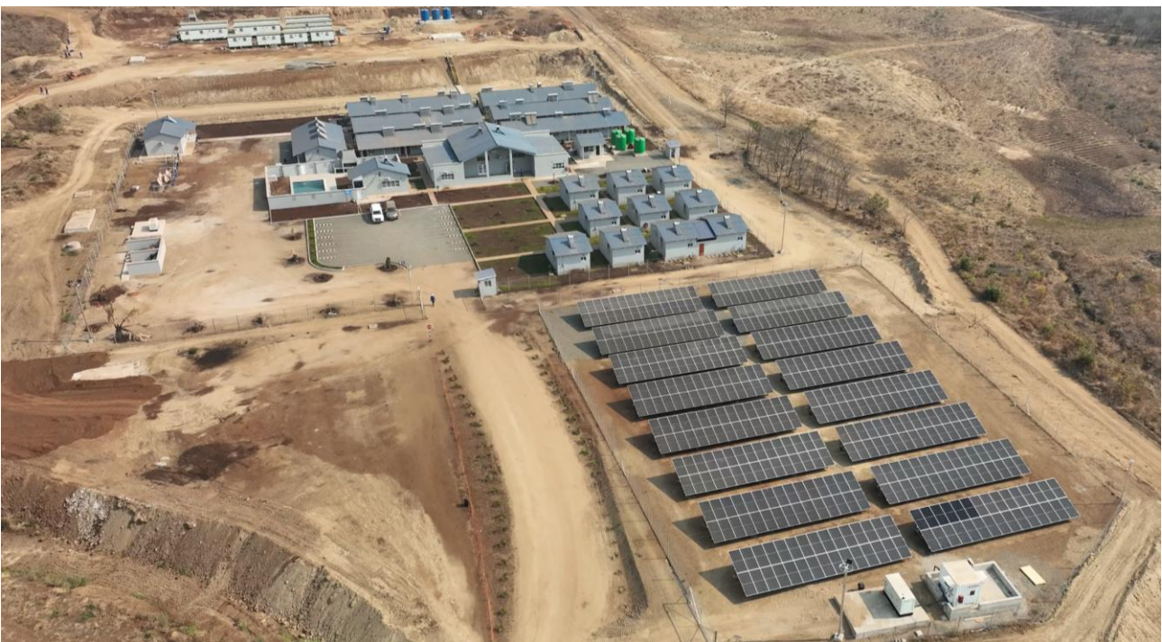
Picture 9. Completed and fully operational Tipume Accommodation Camp and solar installation, supporting the site workforce
