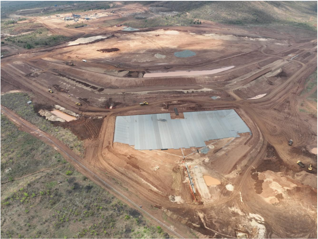
Picture 8. Kangankunde tailings storage facility with bulk earthworks complete
