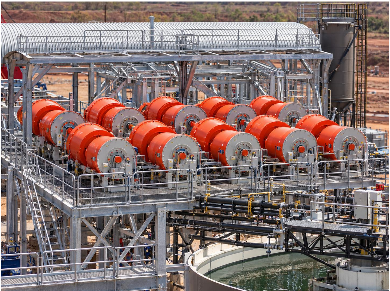
Picture 4. Installation works at Kangankunde process plant
