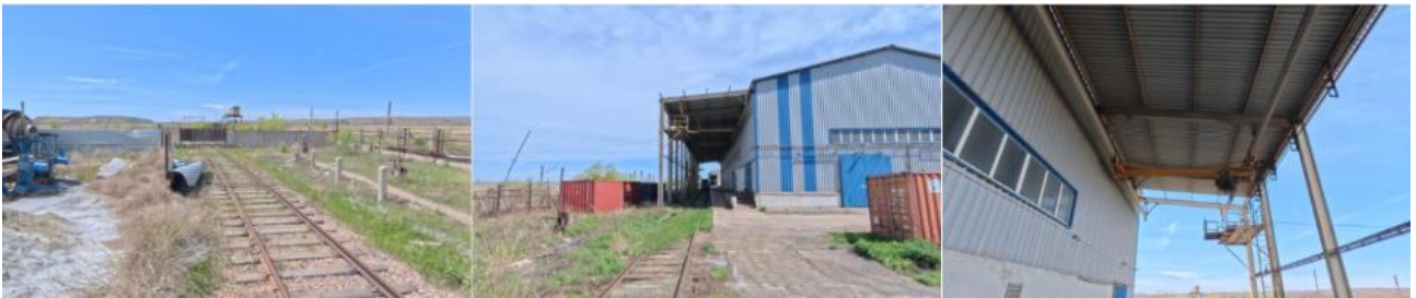
Picture 15. Rail siding and rail car unloading infrastructure at the SARECO Facility
