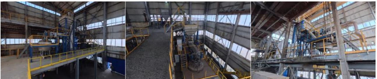
Picture 16. Additional views of the existing SARECO MREC Facility and associated infrastructure.
