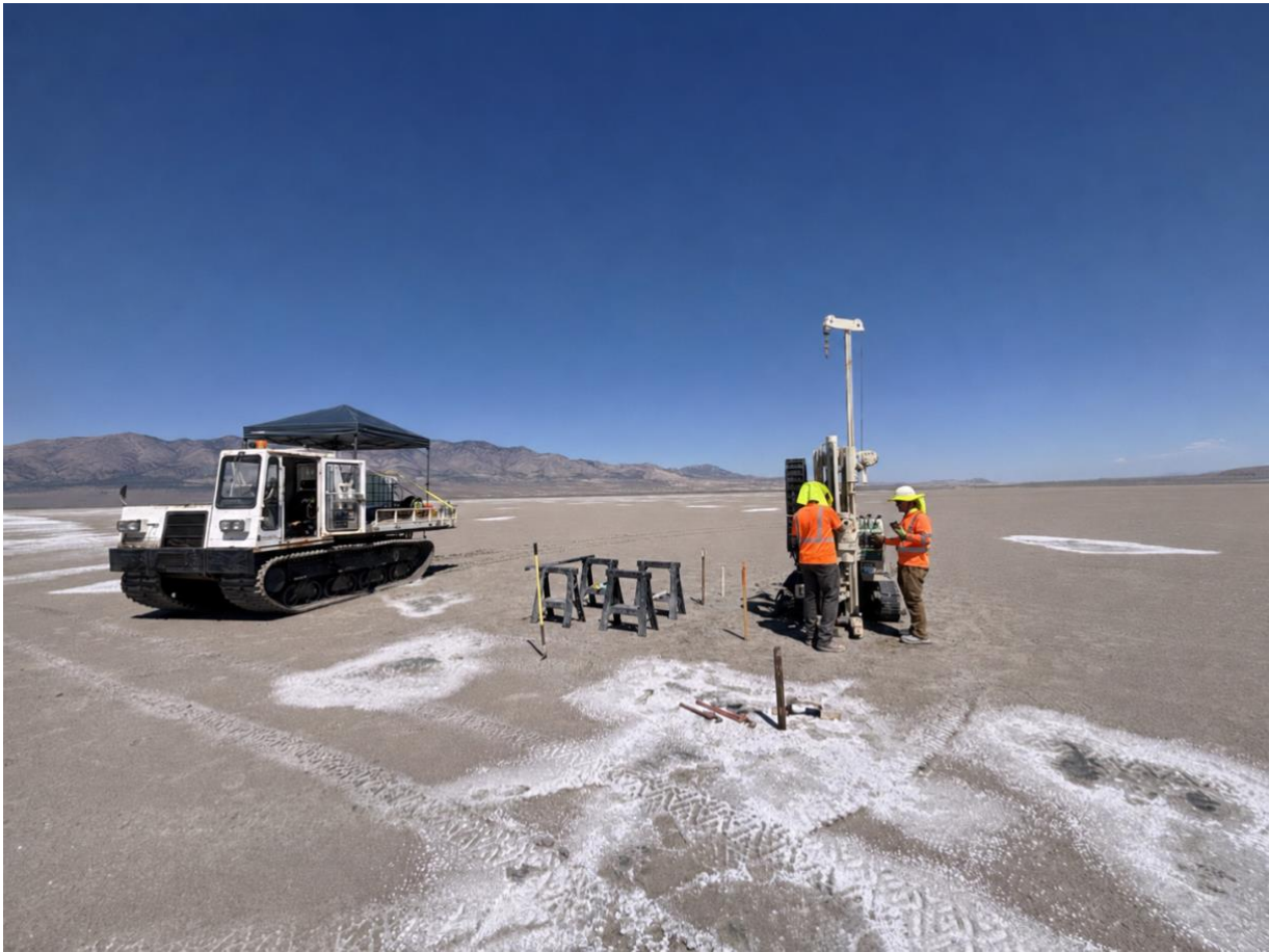
Figure 1: Drilling of Upper Aquifer using a Direct Push Rig at White Plains Lithium Brine Project
