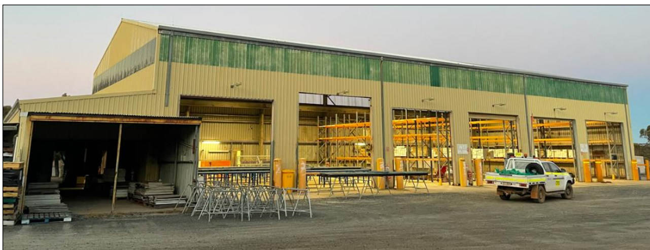
Figure 19: Foster Mine workshop
