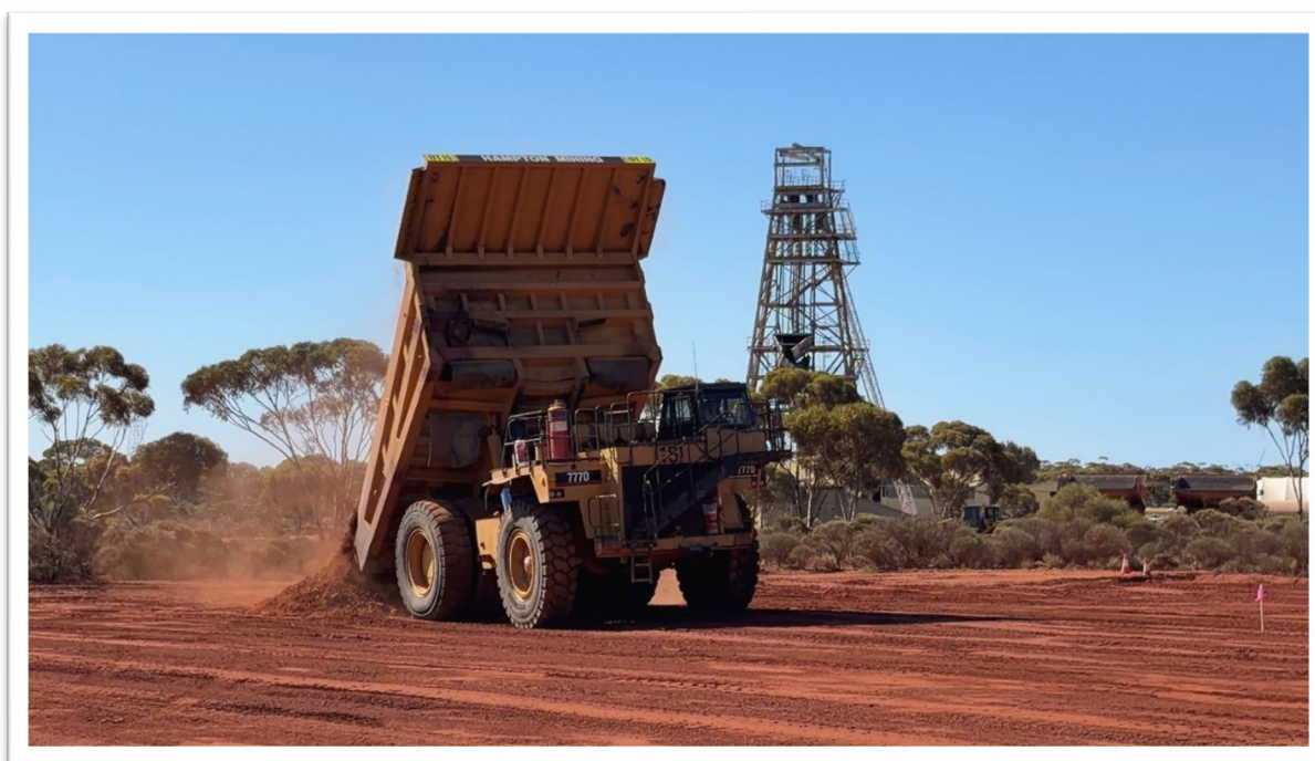
Dumping of first Lady Herial open pit ore on the ROM pad, just 400m to the northwest of Hustler, with the historical Foster nickel mine headframe in the background
