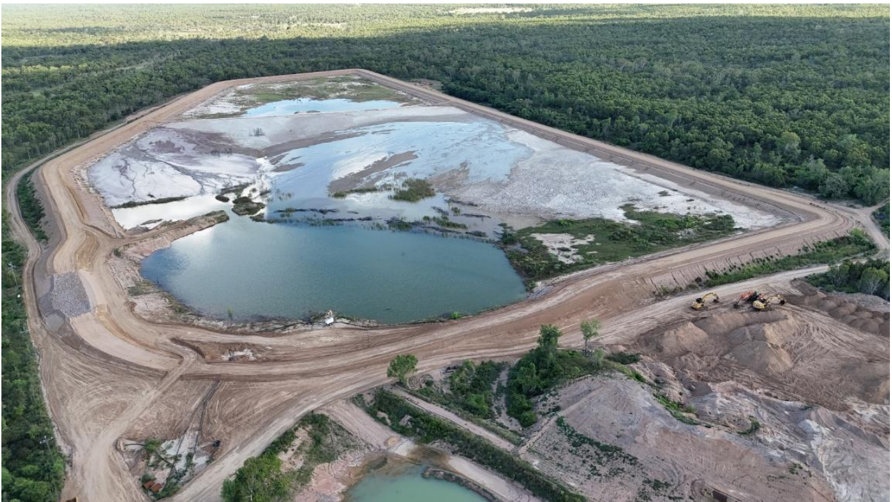
Figure 7: Current TSF with Stage 3 – 2.5m Lift Completed
