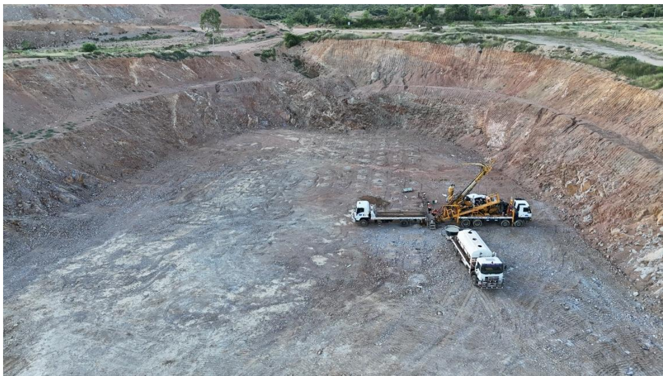
Figure 5: Test Hole Drilling at Blackjack South pit
