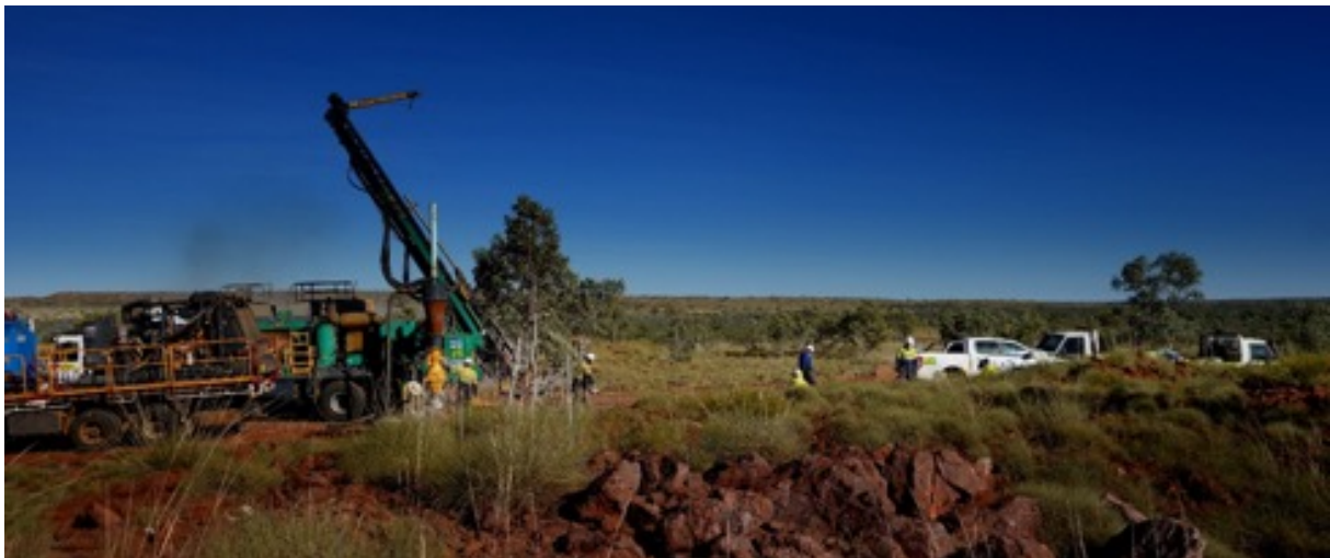
Figure 3 - Initial results from the second phase RC drilling are expected at end of the September quarter, pending laboratory capacity.
