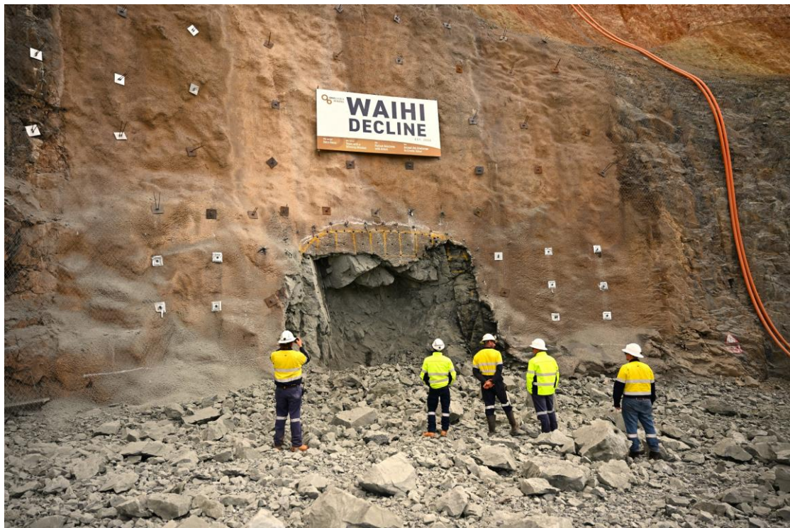
Figure 3 - Inspection of the first cut, Waihi Portal
