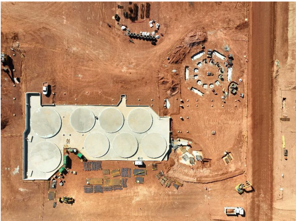
Figure 5– New process plant – Leach tank footing works
