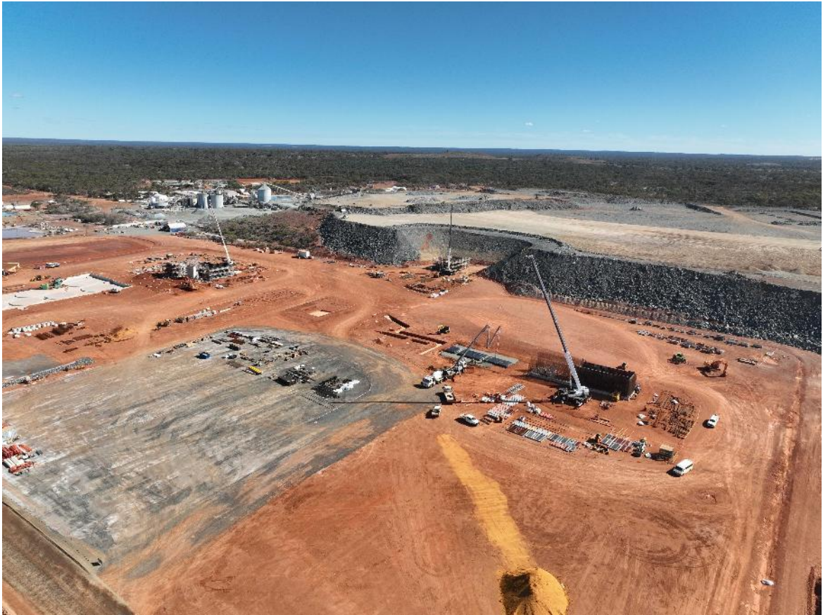
Figure 2 – New process plant works. Background shows existing Davyhurst 1.2 Mtpa processing plant and the enhanced ROM pad.
