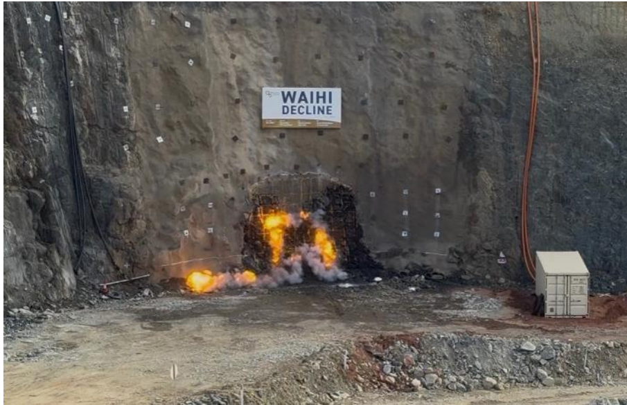
Figure 7 – Waihi Decline portal firing
