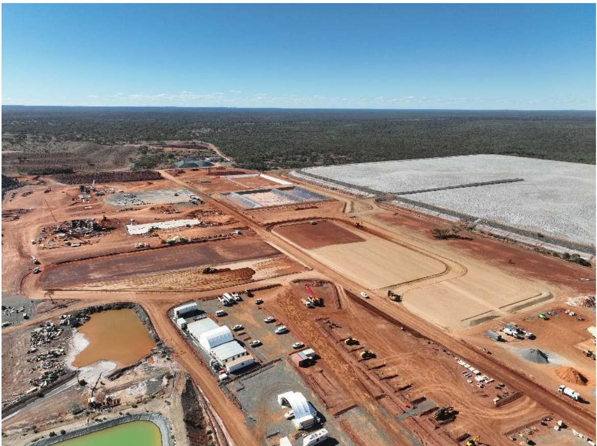
Figure 3– New process plant – general site works
