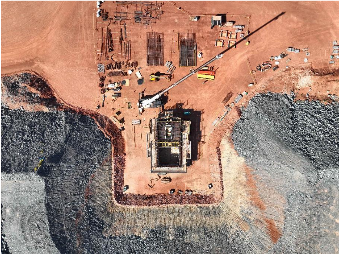
Figure 4– New process plant – Crusher construction
