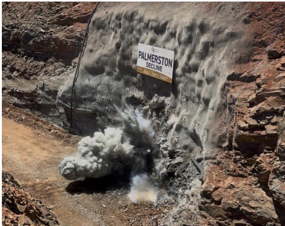
Figure 8– Palmerston Decline portal firing, for access to Sand King North
