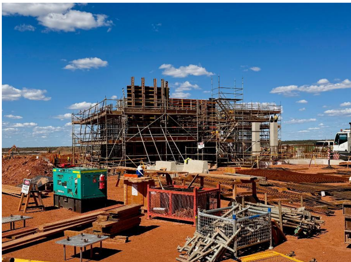
Figure 6– New process plant – mill construction works
