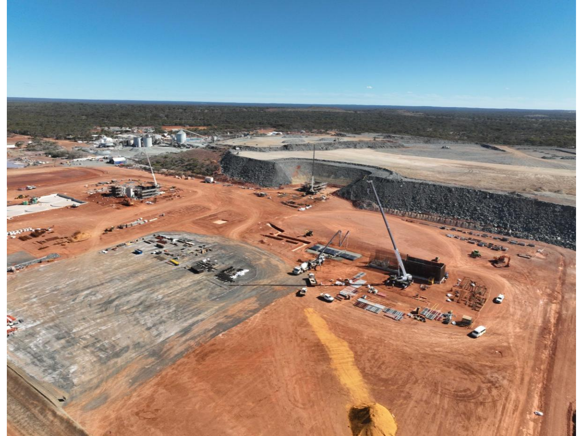
Construction underway of the new processing plant, located next to the existing Davyhurst Mill
