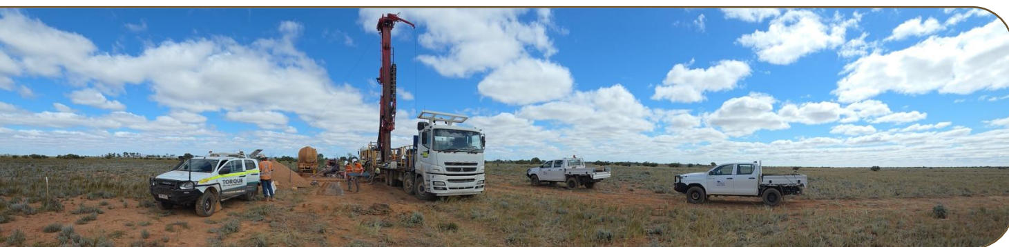
Photo: Drilling underway at the Frome Project (September 2026)
