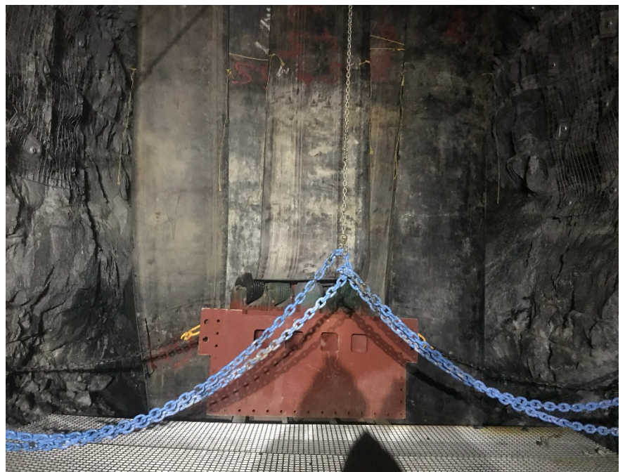
Figure 5: safety curtains installed prior to reamer wing extensions being installed
