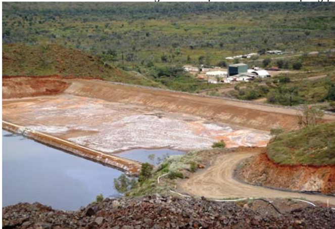
Photo 1: Savannah tailings storage facility and the three metre embankment lift
