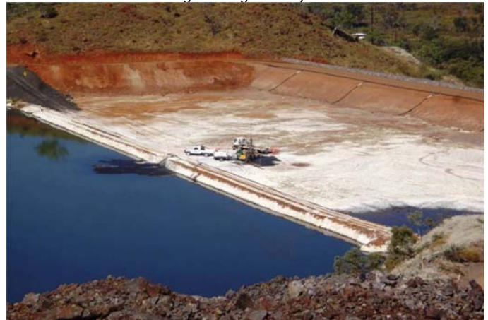
Photo 2: Drilling of new monitoring bore holes on the tailings storage facility
