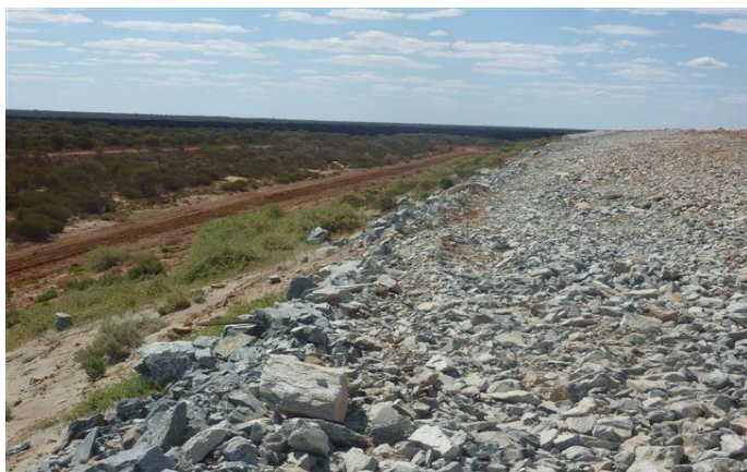
Photos 1 and 2: Capping work on the Gidgee TSF
