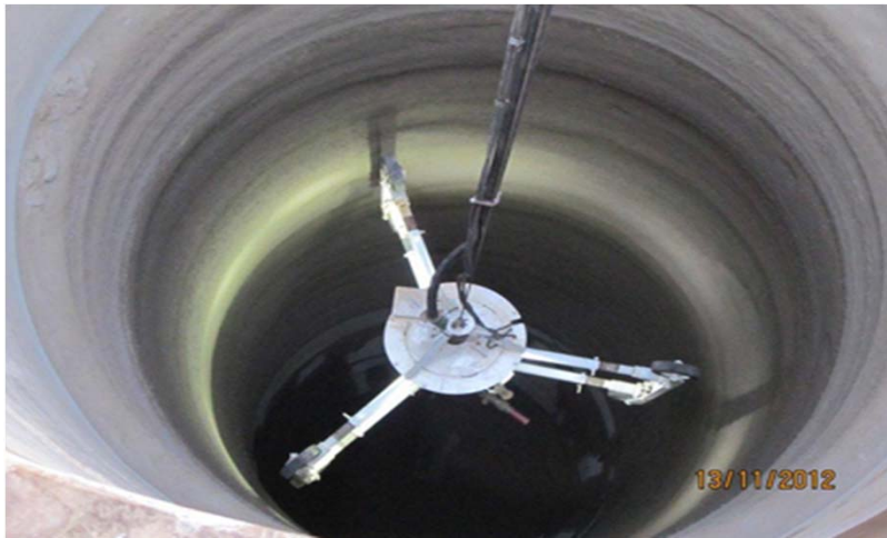
← Shotcreting vent shaft
