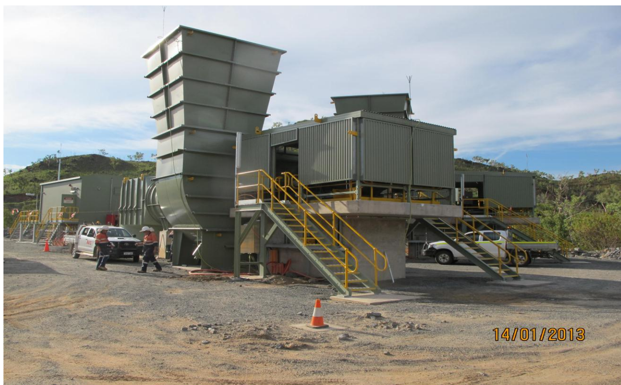
Photo 1: Savannah surface fan and associated infrastructure
